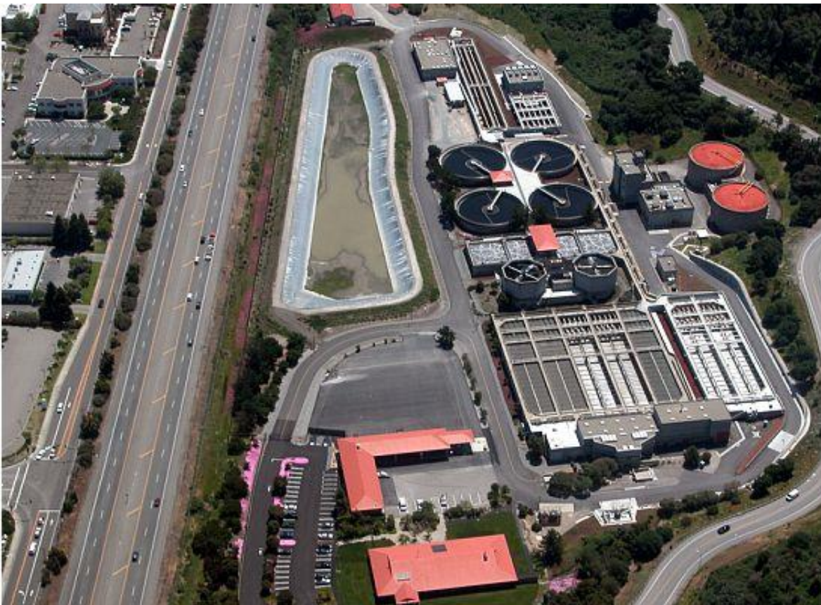
(Clockwise upper left to right): Effluent Storage Pond, Maintenance Annex (red roof behind the pond), Chlorination/Dechlorination Building, Chlorine Contact Tanks, Effluent Pump Station, Secondary Clarifiers, Solids Handling Building, Digesters and Digester Building, Aeration Tanks, Biotowers, Primary Clarifiers and Blending Channel, Grit Building, and Headworks. The two orange roofed building in the lower center are the Maintenance Building (top) and the Administration Building (bottom).
