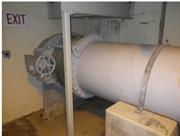
Primary Effluent Pipe emerging into gallery
