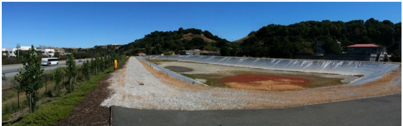
Effluent Storage Pond
