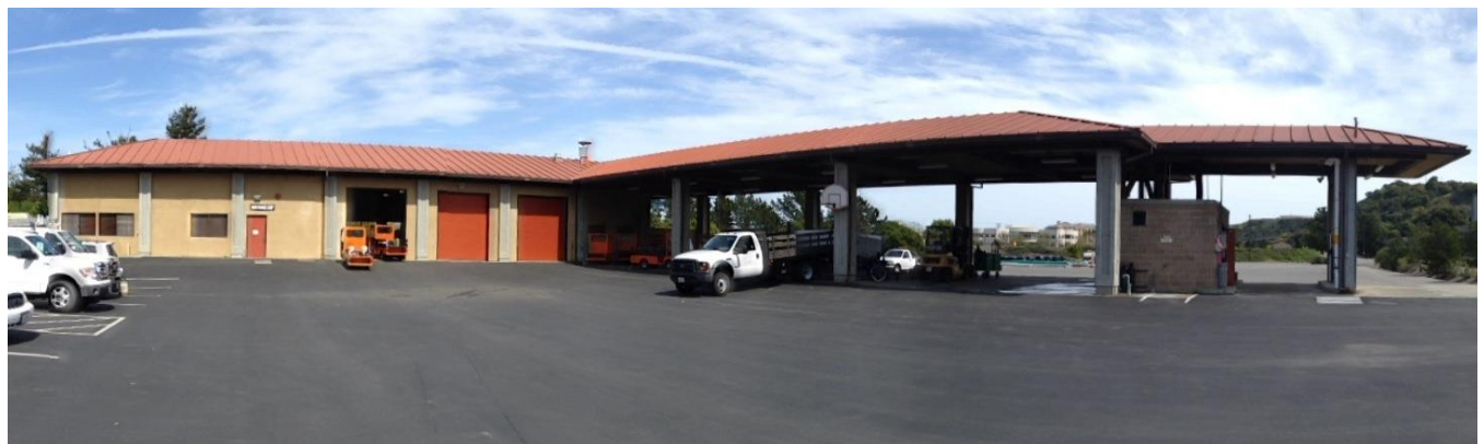
Maintenance Building with standing seam metal roofs.
