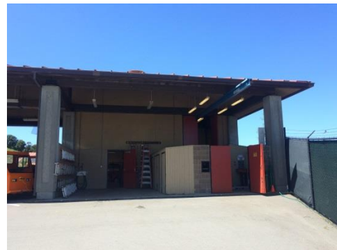
Area to be enclosed for additional storage
