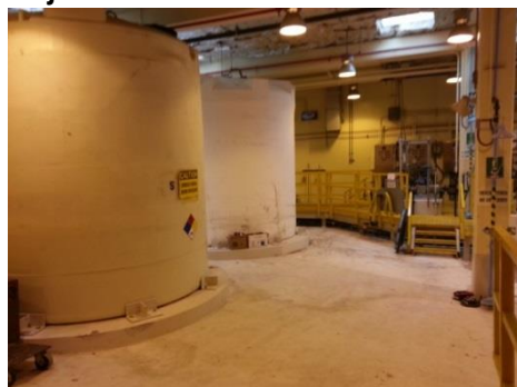
Hypochlorite room showing floor damage
