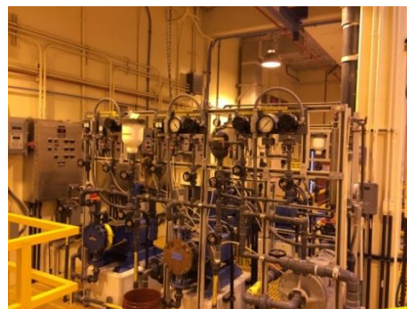
Hypochlorite room pumps and piping
