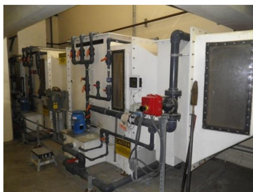
Odor control scrubbers, with air handlers, two views.
