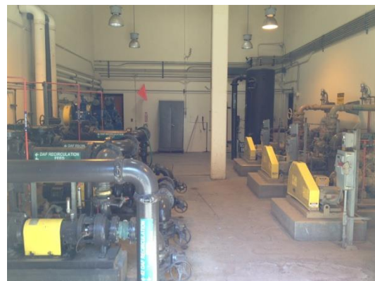
DAF Equipment Room
