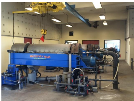
Existing Centrifuges
