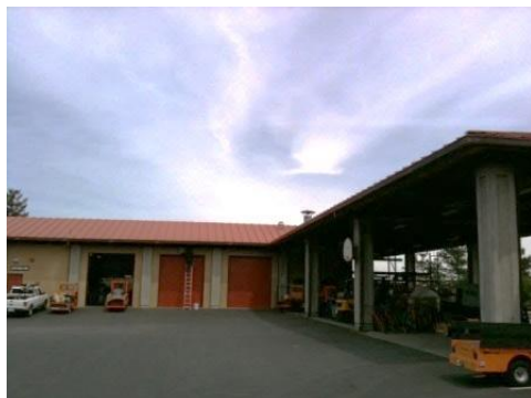
Maintenance Building and Covered Portico
